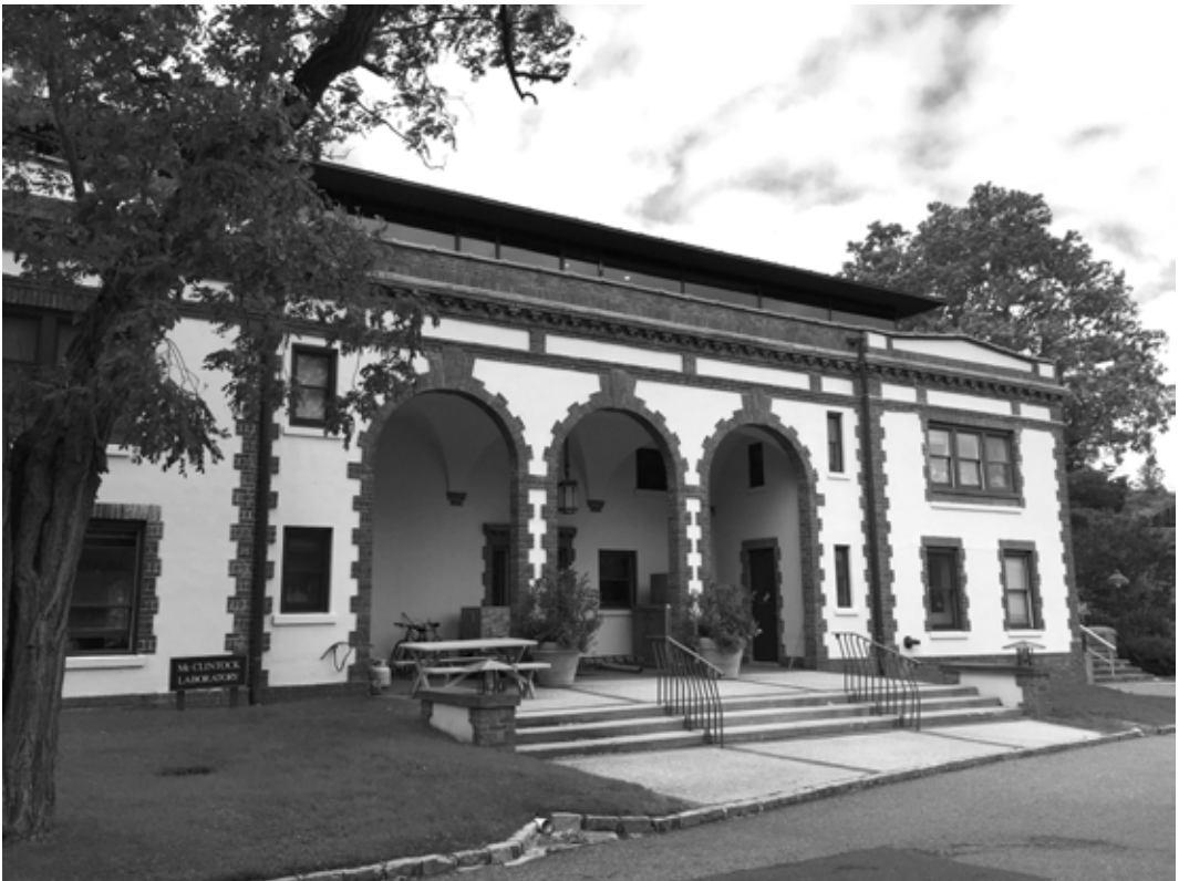
Fig. 1 - The former Carnegie Institution Building at CSHL. Photograph by S. Kaji-O'Grady.
