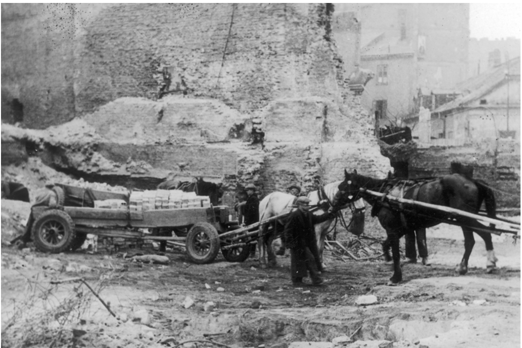
Fig. 2 - Brick salvaging in the ruins of the central Warsaw, 1948. Socialist Press Agency, National Press Agency, National Digital Archive.
