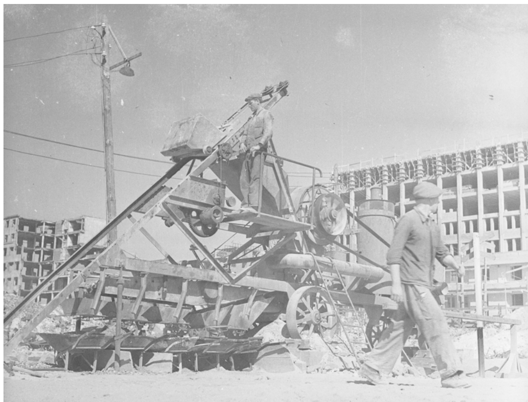
Fig. 6 - Rubble crusher and sorter in operation in central Warsaw, 1948. It is one part of the larger mechanical assembly producing air bricks, eighteen of which were acquired in Switzerland in 1946. Military Photographic Agency, National Digital Archive (WAF, 1948).
