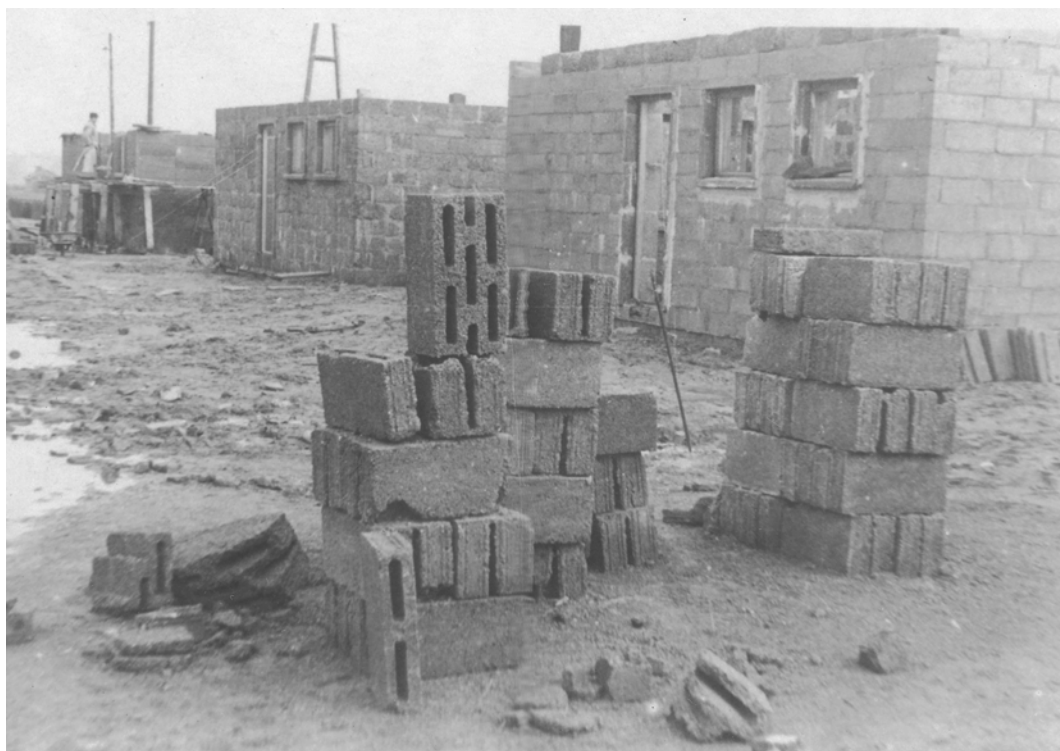
Fig. 5 - Air bricks made from a mix of crushed-rubble aggregates and sands with cement and water, Warsaw, 1948. Socialist Press Agency, National Digital Archive.
